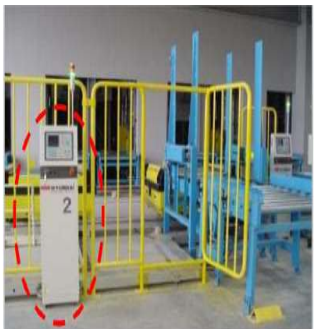
▶ Stacker Crane Operation Panel
