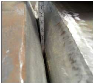
Root gap & cleaning condition check
